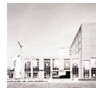
ARVENA PARK Bauphase
