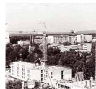
ARVENA PARK Bauphase
